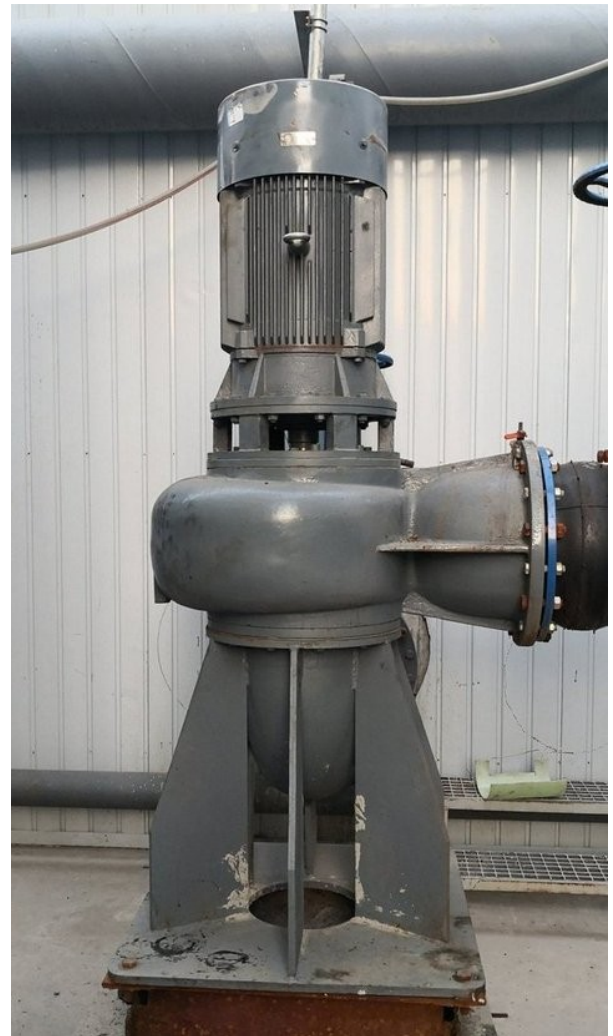
Above, a large LW pump installed with suction inlet arranged at 90 degrees to outlet.
